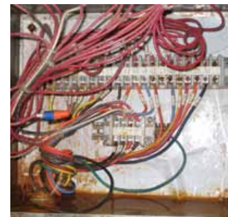
Water accumulation in electrical cabinet
