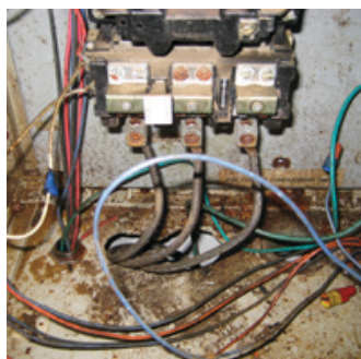
Corrosion leads to premature component failure
