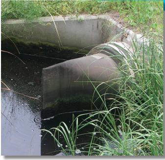
Detail of the *ProFlex™* Slip-on Rubber Check Valve; Style 730
