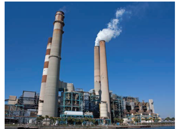
Obsolete PV09 pumps are common in the power generation industry, particularly in EHC systems controlling aspects of GE Steam Turbines.
